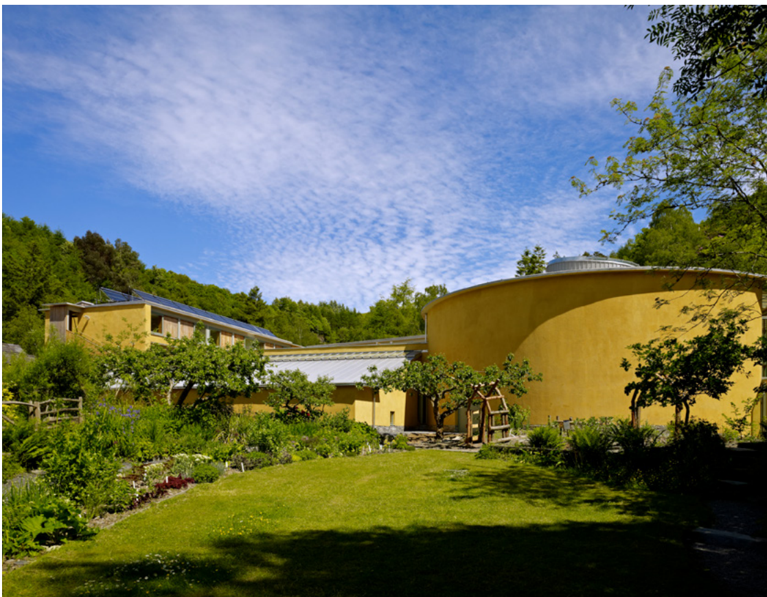
The circular building on the right is the 7.2 metres high Sheppard Theatre, which has one of the highest rammed-earth walls in the UK.
